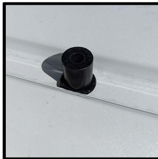
Next apply a liberal amount of silicon over the plusnuts the place the spacers on top
