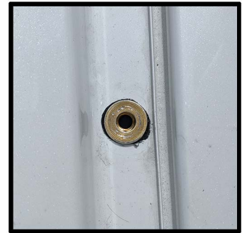
Plusnut placed in roof
